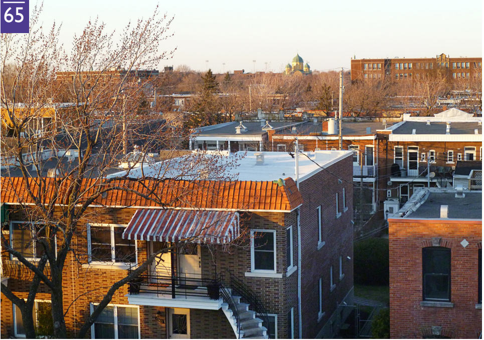
Figure 15: The image above shows a residential building with a cool roof in Rosemont-La Petite-Patrie (Source: Arrondissement Rosemont-La Petite-Patrie)
