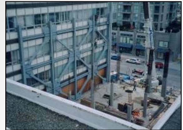
Lion's Gate Hospital North Vancouver
