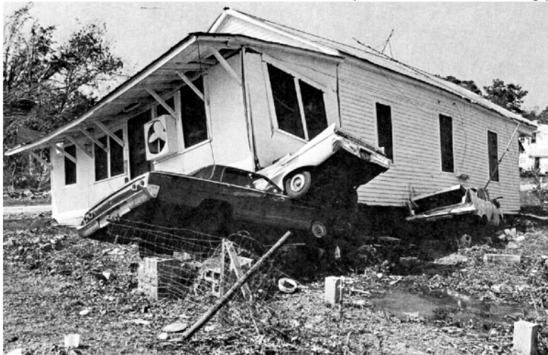
House At Rest On Top of Cars
