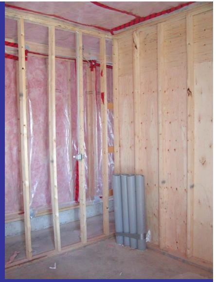
Control Building test wall panels for mould and moisture penetration studies
