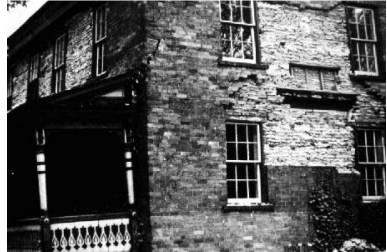
Masonry damage
