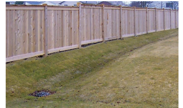
Rear-yard swales direct flows to a catch basin in this image. Rear-yard catch basins and swales shouldn't be covered or filled in with backyard sheds, fences or other structures, and rear-yard catch basins should be kept clear to reduce backyard flooding.
