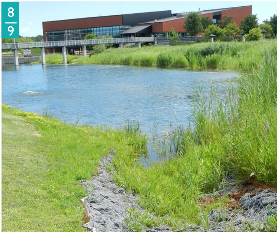
Figure 2: Boucherville won awards for installing wet and dry ponds to retain stormwater in a new development.
