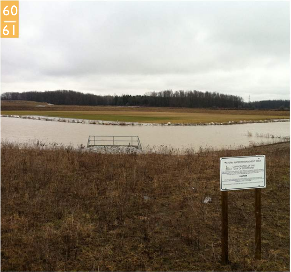
Figure 16 : Stormwater management pond built in Stratford to accommodate surcharging of local systems. (Source: City of Stratford)
