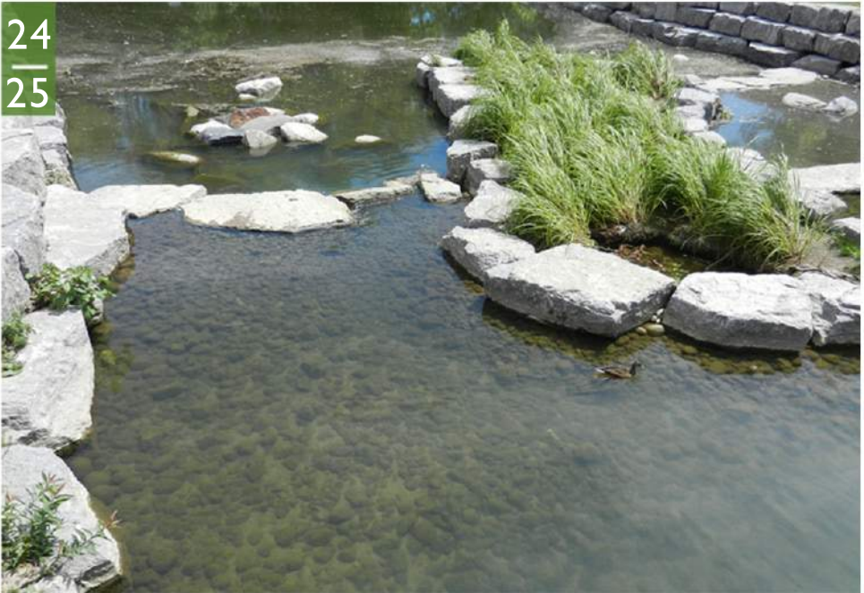
Figure 6 : The Victoria Park Lake Improvement project includes a new sediment forebay. It is designed as an initial storage area to trap and settle out sediment and heavy pollutants before they reach the main basin. (Source: ICLR)
