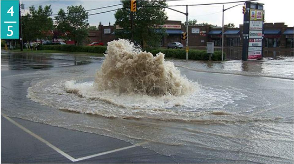
Figure 1: Extreme rainfall event in Ottawa in 2006 causing sewer overflow. (Source: City of Ottawa)
