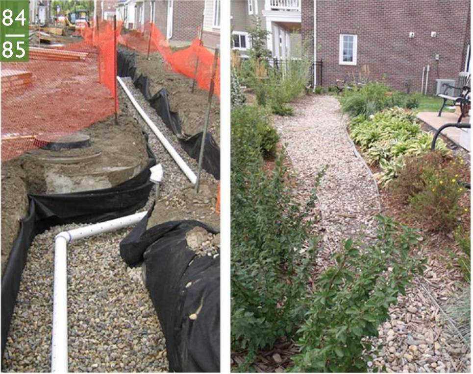
Figure 25 : The pictures above show an infiltration trench built in the Currie Barracks Brownfield re-development project. An infiltration trench is an excavated trench backfilled with stones to create a narrow underground reservoir. Stormwater runoff diverted into the trench drains from the bottom of the trench into the subsoil and eventually to the water table.
