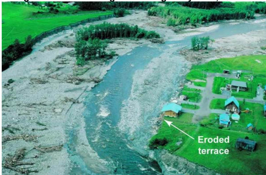
Figure 2: Flood Damage in the Saguenay Area, Quebec
