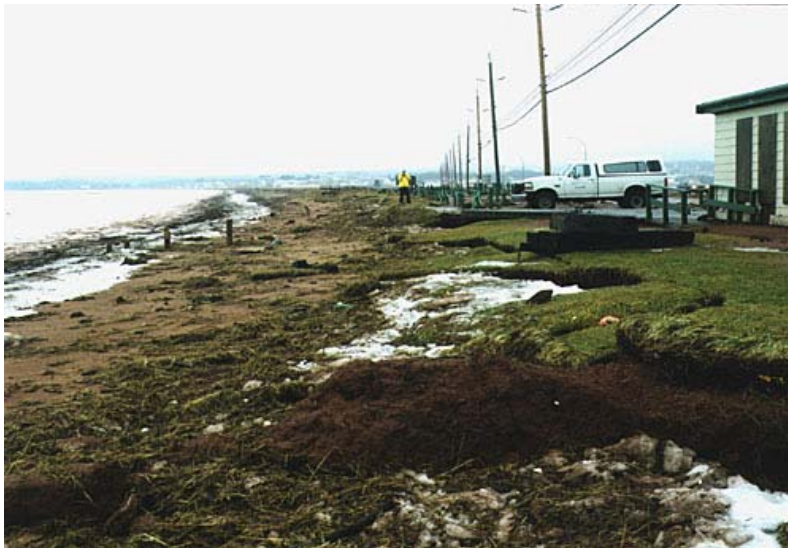
Figure 3: Wave Damage at Souris, Prince Edward Island
