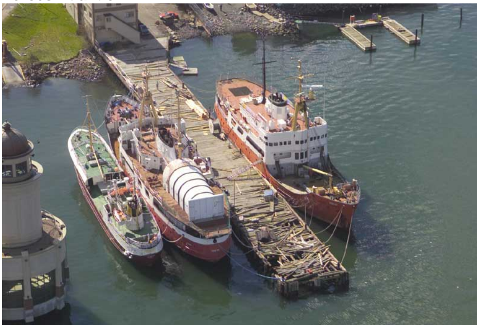
Figure 1: Storm surge causes wharf damage in Halifax Harbour - Maritime Forces Atlantic
