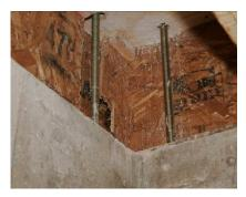
The frame of the home is bolted to the foundation.
