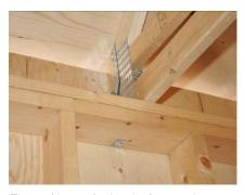
The roof is attached to the frame using special clips.
