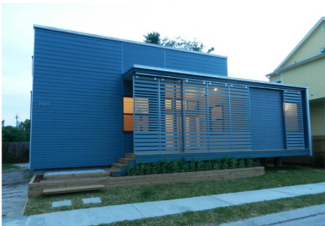
Figure 5: Tulane URBANbuild housing prototype. Source: www.tulaneurbanbuild.com
