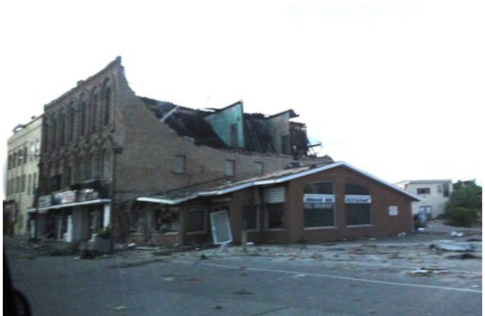
Damage from the Goderich tornado, August 2011.
