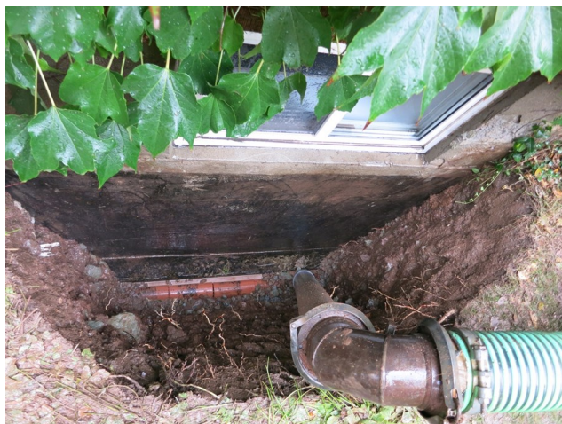
Window well installation in the Burlington home, November 2014.
