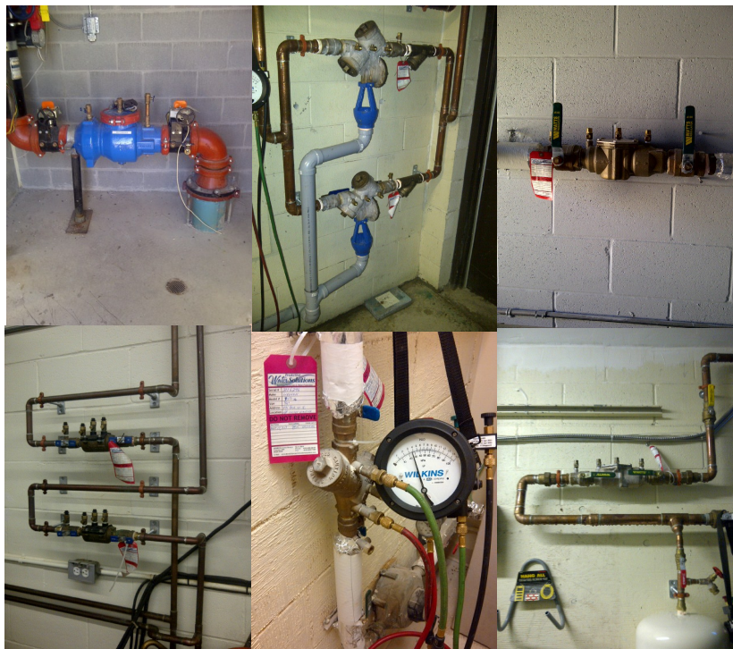
A montage of various types and styles of backflow preventer or backflow prevention device, courtesy ProActive Water Solutions Inc. www.proactivewatersolutions.com
