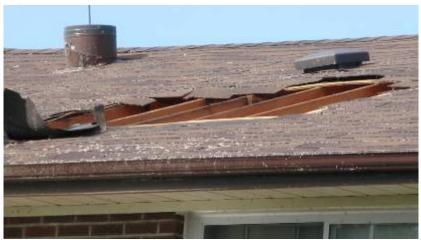
Sheathing failure caused by inadequate hold-down strength, likely missing nails or deteriorated materials, in Vaughan, Ontario. durability within the intended life span, and (iv) potentially inappropriate prescriptive design standards which may overestimate the capacity or underestimate the load.
