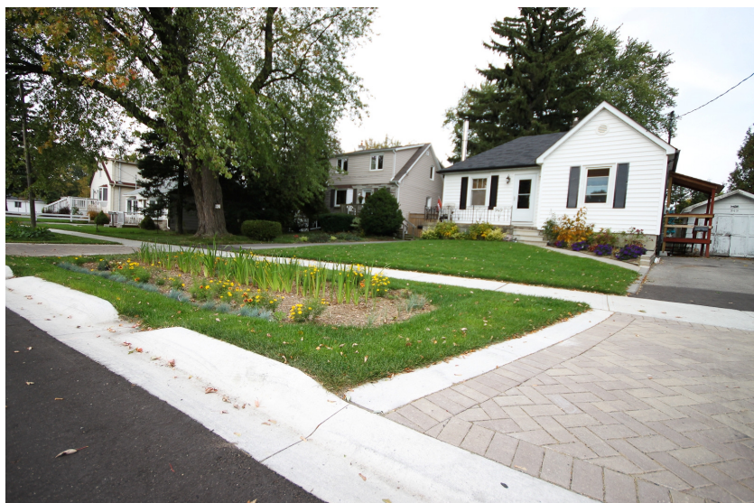
A “green street” in the Lakeview neighborhood of Mississauga incorporates permeable paver driveways, curb cuts and bioretention or “rain” gardens to treat rainfall and urban runoff where it falls.
