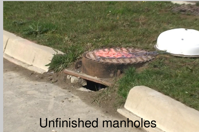
Catchbasins not yet commissioned & covered in geotextile
