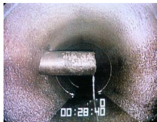
Sewer Protrusion
