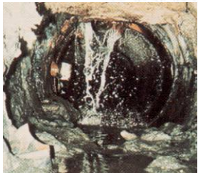
Cracked Sewer
