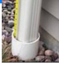
Downspout to storm sewer
