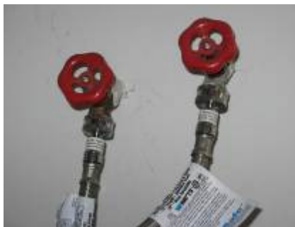
Armoured washing machine hoses can prevent water damage should the common rubber hoses fail. These inexpensive hoses should also be used on dish-washers, sinks and toilets.
