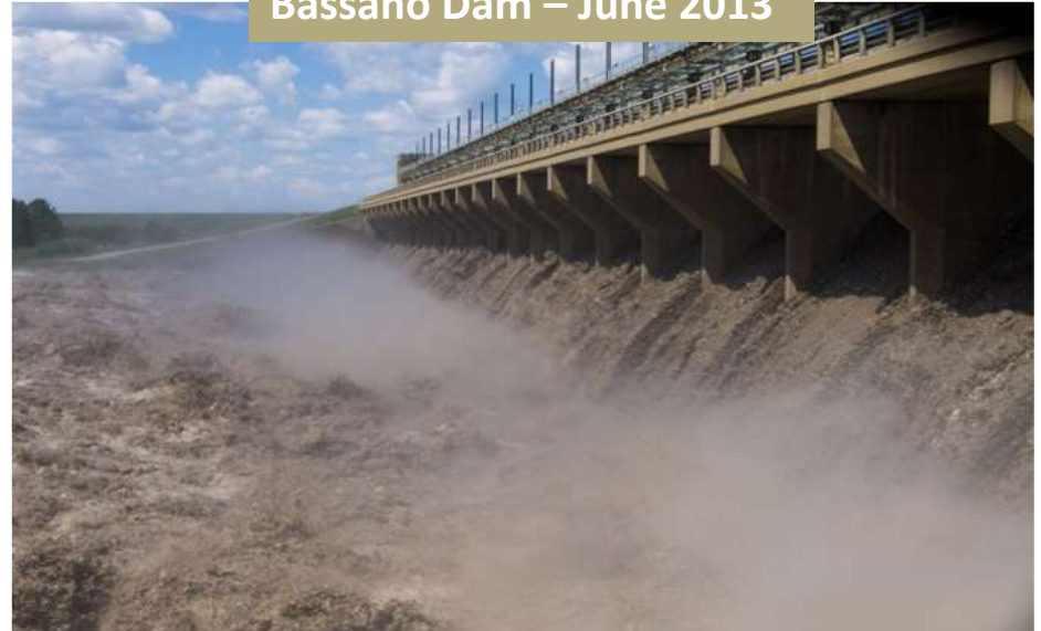
Bassano Dam – June 2013
