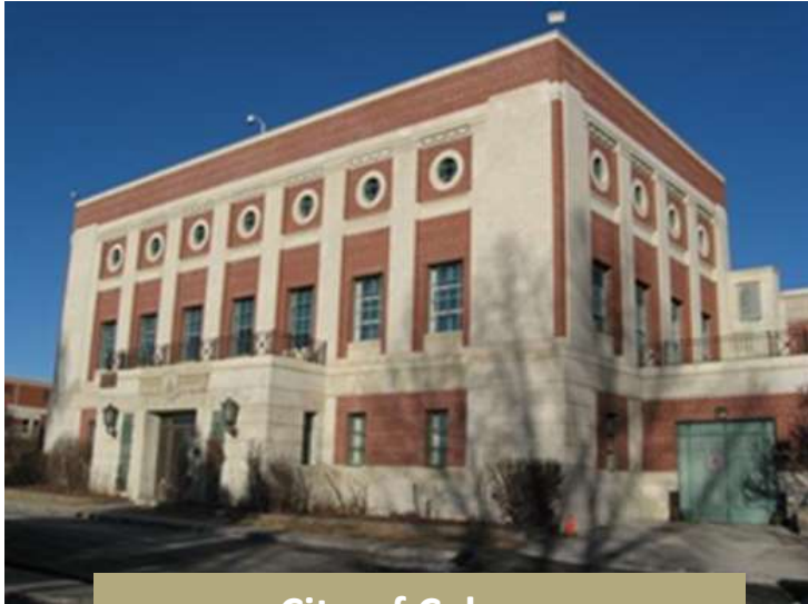
City of Calgary Glenmore Reservoir Water Treatment Plant
