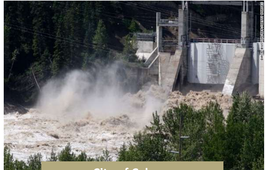
City of Calgary Bears paw Water Treatment Plant during 2013 Flood
