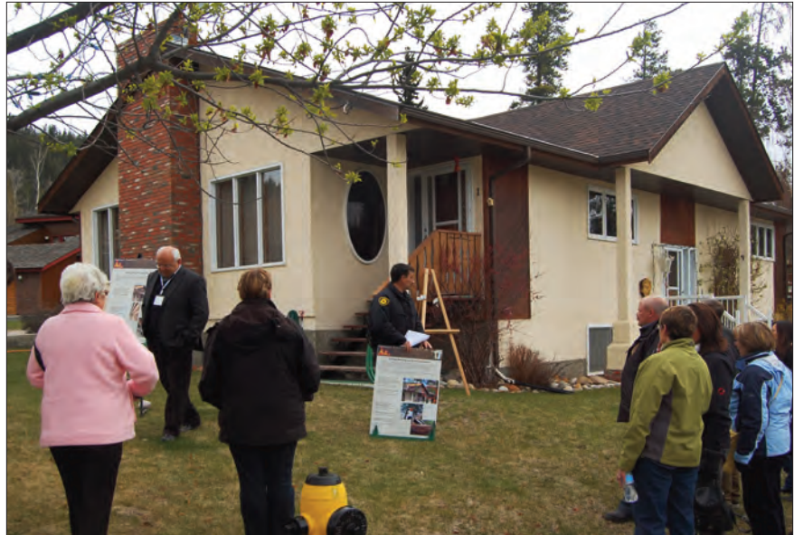
Home in Jasper Alberta retrofitted to protect against wildfires, May, 2010.
