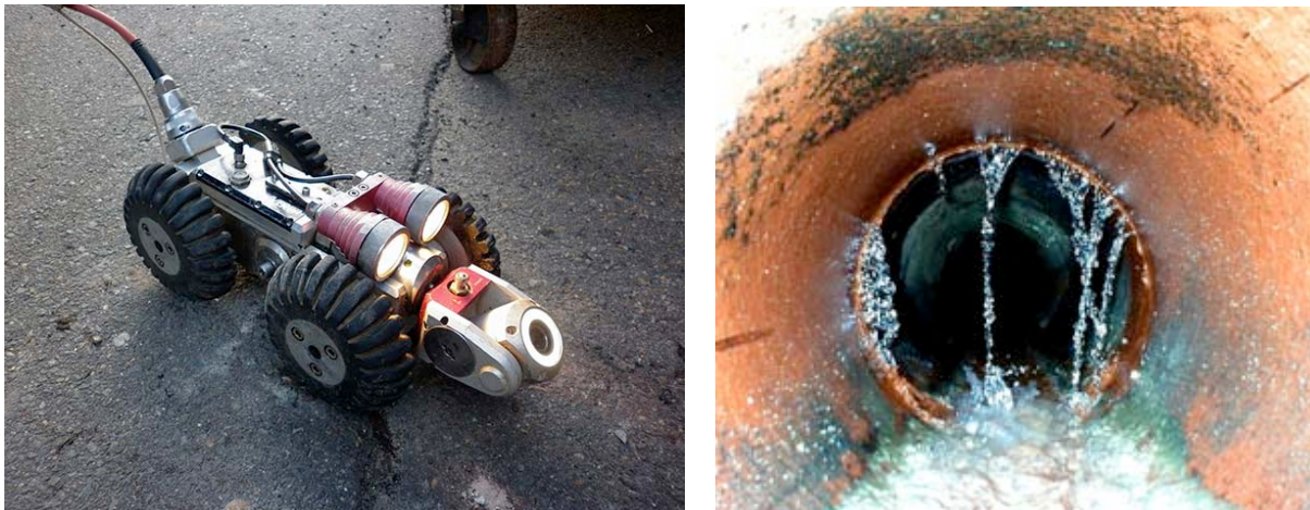
Figure 22. A remote controlled tractor with an articulating closed circuit television (CCTV) camera is able to detect defects such as leaks at joints, as well as any defects or deterioration of materials. [Source: Online Pipe and Cable Locating.]
