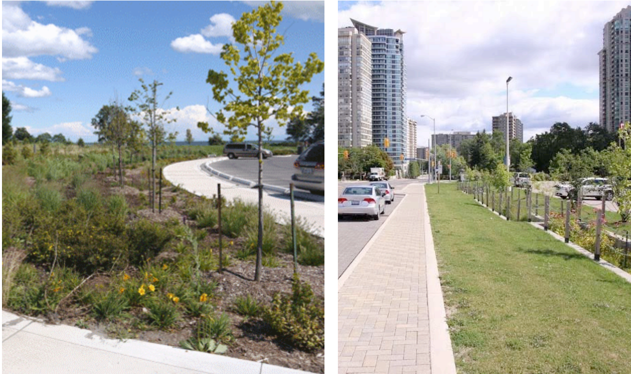
Figure 18. Examples of bioswales used to sequester runoff from a parking lot (left image) and both roadway and parking lot (right image). The detention of runoff manages both stormwater volumes and water quality in aesthetically pleasing landscape features. [Source: Credit Valley Conservation Authority, Ontario.]
