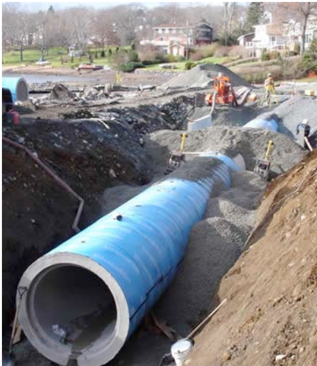
Waterproof membranes over sewer pipes.
