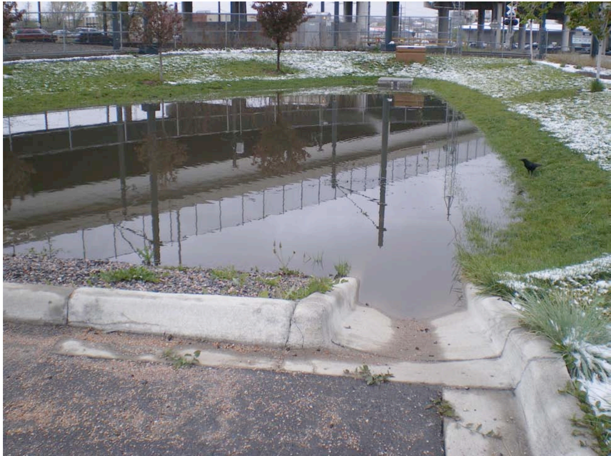
Figure 19. Infiltration basins located away from buried infrastructure may represent preferred low impact development measures in areas where the hydraulic conductivity of the local soils causes infiltration stresses on sanitary sewer pipes and maintenance holes. [Source: Construction Specifier Magazine, Canada.]
