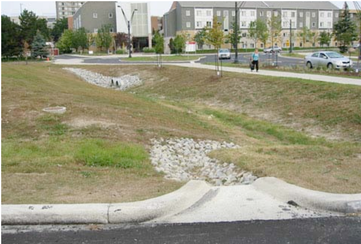
Figure 11. The construction of bioswales is a highly effective low impact development measure for managing stormwater on site. Properly situated, these measures can manage runoff from adjacent hard surfaces, such as roadways and parking lots. [Source: Toronto and Region Conservation Authority]
