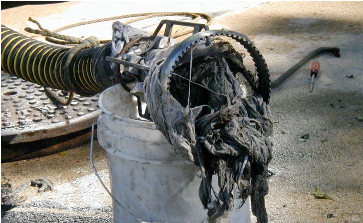
Figure 12. Regular cleaning of sanitary sewers to avoid blockages and backups not only maintains proper performance, but also enables the proper monitoring of infiltration. [Source: Town of Yorkton, Saskatchewan.]
