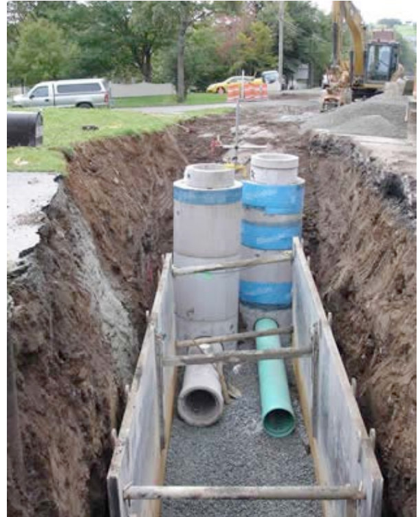
Waterproof membranes at maintenance hole joints.
