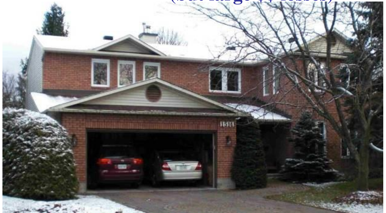
1980s wood frame 2-storey with brick vener
