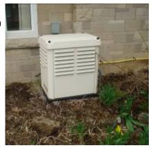
A natural gas-fired generator was installed to ensure that the home's two sump pumps have a dedicated power supply in the event of a disruption.
