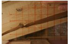
Figure 4: Example of a toenail roof to wall connection in the house where the nail has split the wood and offers very little hold down force.
