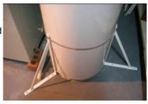
The home's water heater was fastened to the floor to prevent it from toppling over in the event of an earthquake or other disturbance. This prevents the gas line from severing, causing an explosion and fire, and also prevents water damage.
