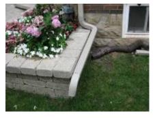
Downspouts were extended to convey rainwater away from the foundation.
