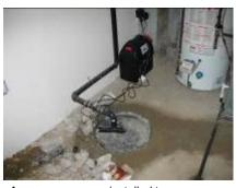
A sump-pump was installed to convey rainwater out of the weeping tiles, bring it to the surface of the lot, and pump it onto the lawn (away from the foundation) in order to keep excess water out of the municipal system.
