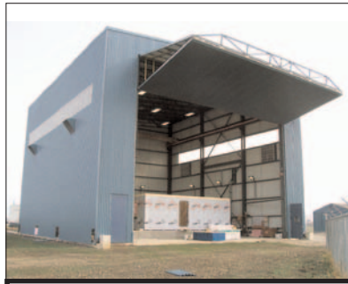
Main building covering the first house test specimen, under construction
