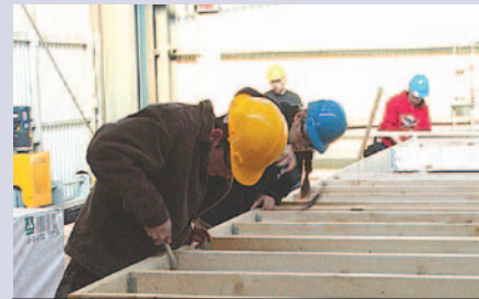
Fanshawe College students framing floor of first full-scale test specimen
