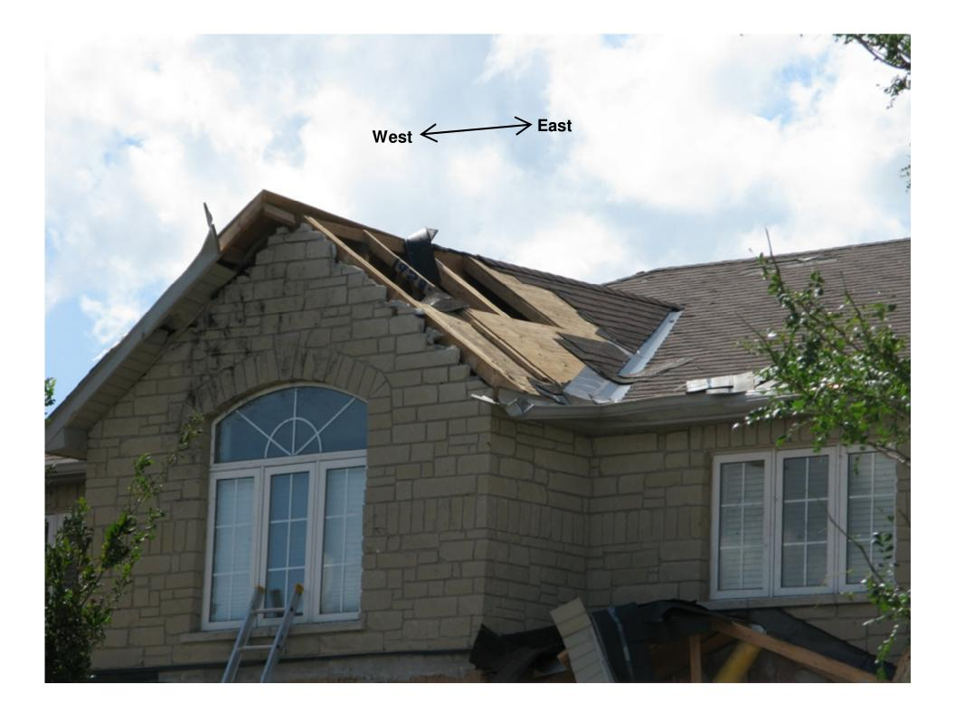
Sheathing without enough fasteners ... not even the shingles came off here
