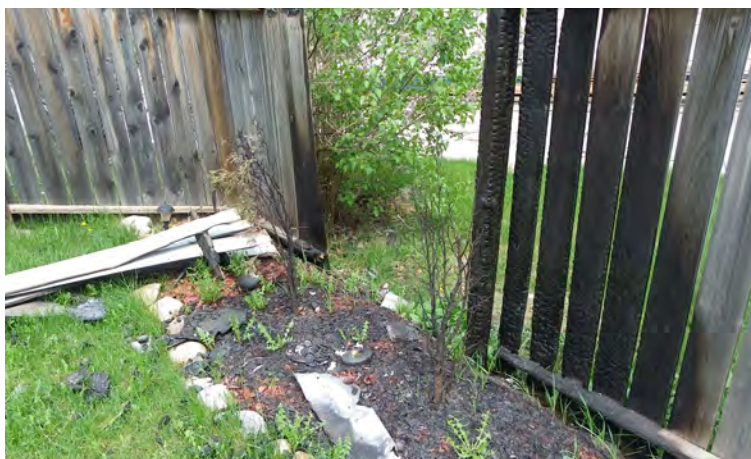
Figure 5-6: Combustible wood chip/bark mulch was easily kindled by embers and readily spread fire
