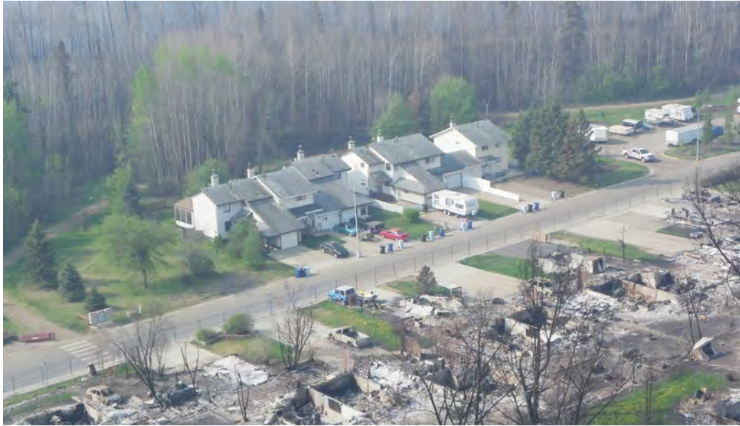
Figure 3-1: Investigations focused on homes near the 'front line' adjacent to forested areas
