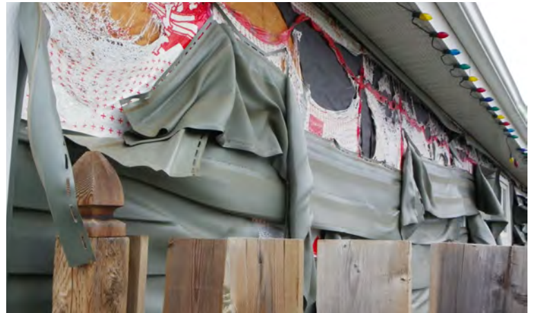
Figure 5-1: A significant proportion of Fort McMurray homes had exterior vinyl siding
