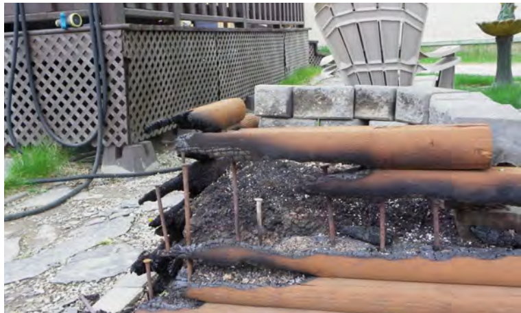
Figure 5-8: Landscaping timbers smoldered persistently and spread fire into contact with structures
