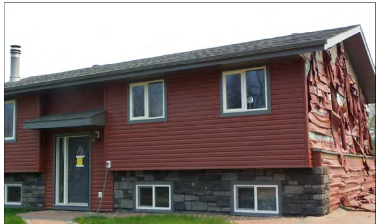
Figure 4-5: Homes surviving extreme exposure had uniformly low vegetation/fuel hazard within 30m
