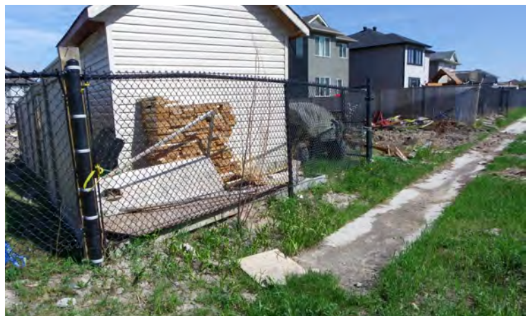
Figure 5-4: Vulnerable outbuildings were a heat source capable of igniting homes
