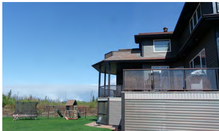
Figure 5-2: Example of decks exhibiting low-risk features in area exposed to high ember density
