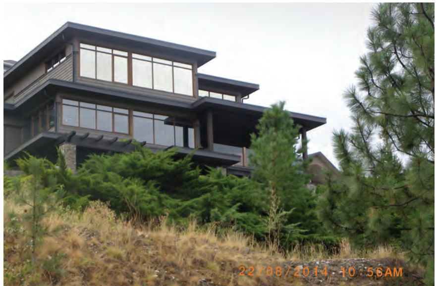
Figure 4-9: Topography compounds other hazards and is difficult to mitigate.
