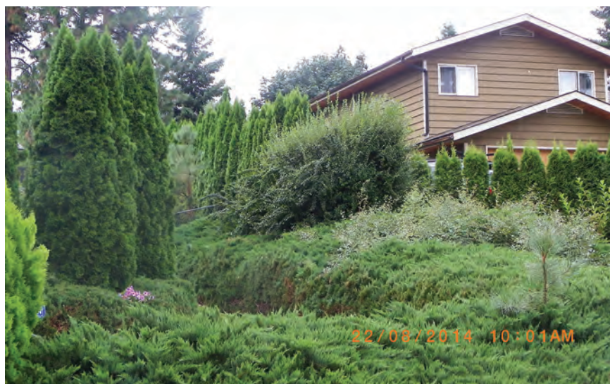
Figure 4-3: Non-conforming vegetation/fuel accounted for 58% of all wildfire hazards.
