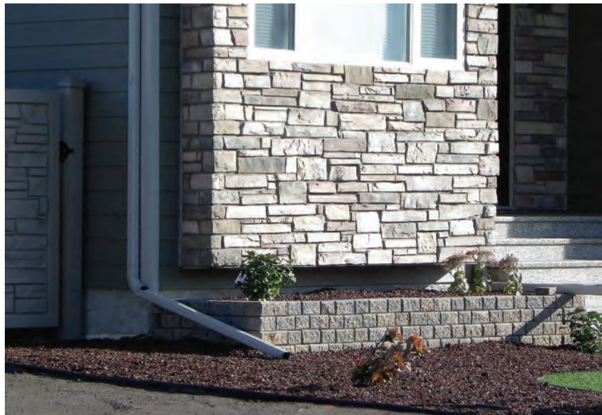
Figure 4-5: Fire resistant siding and windows reduced wildfire hazard.
