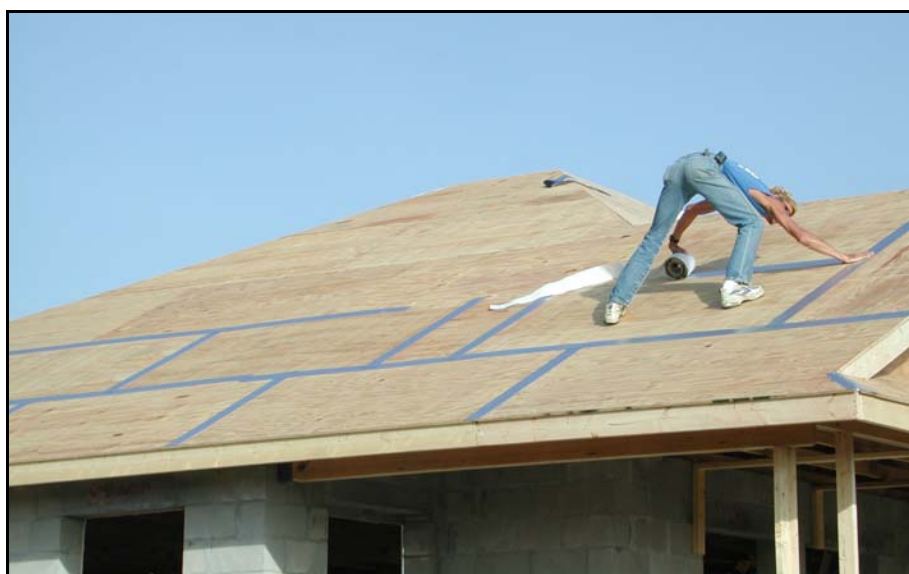
Figure 3.19: Installation of secondary water resistance using self-adhering strips.
