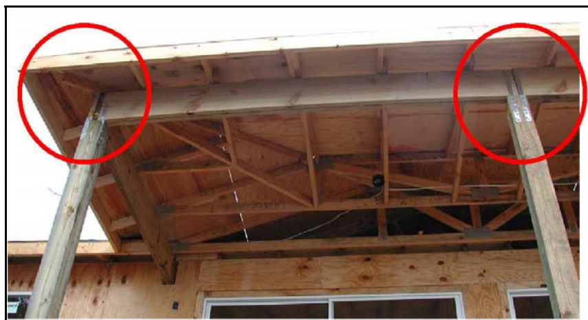
Figure 3.12: Strapping of top of porch column to supporting beam.
