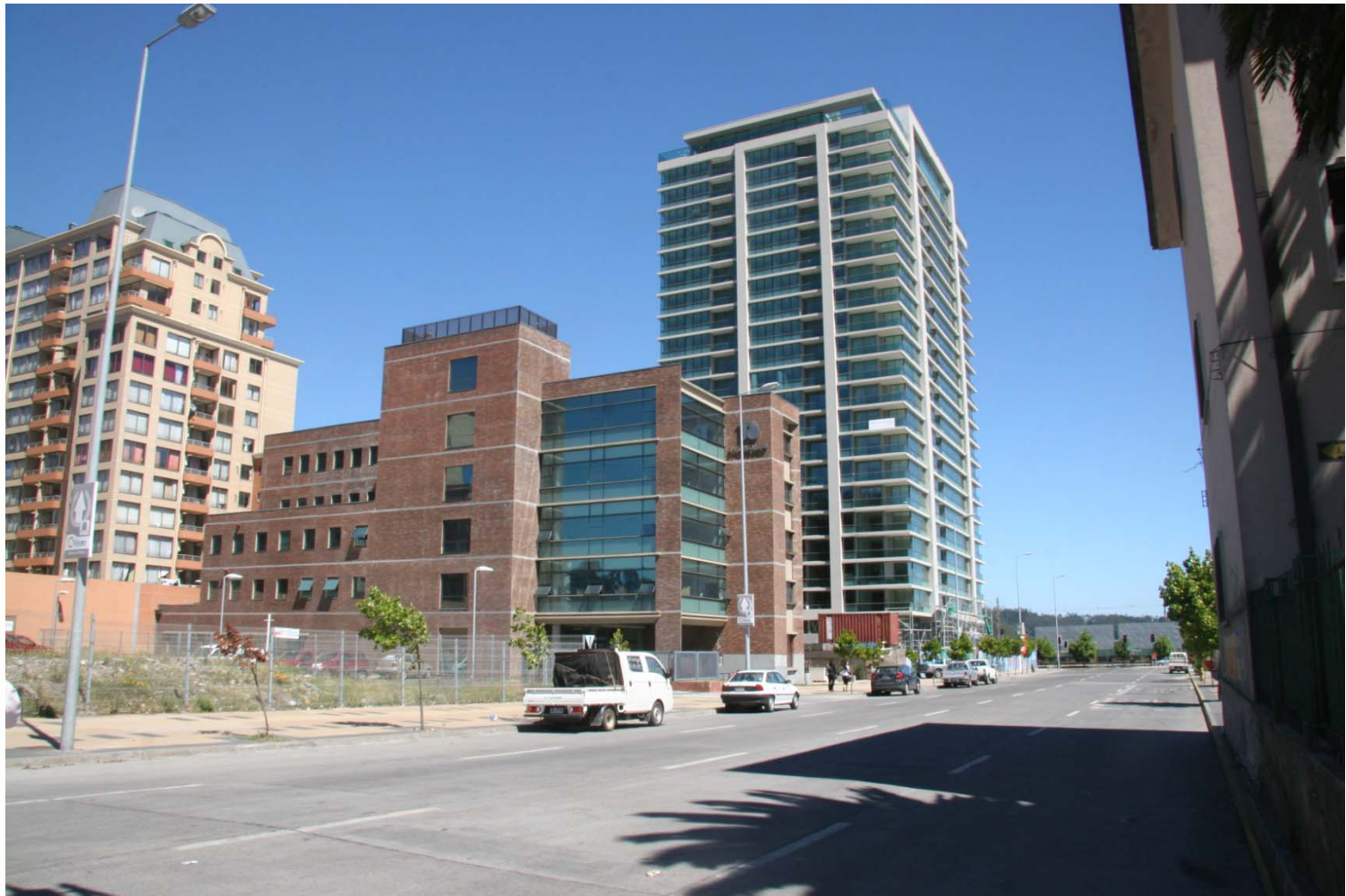
Examples of buildings that survived this earthquake
