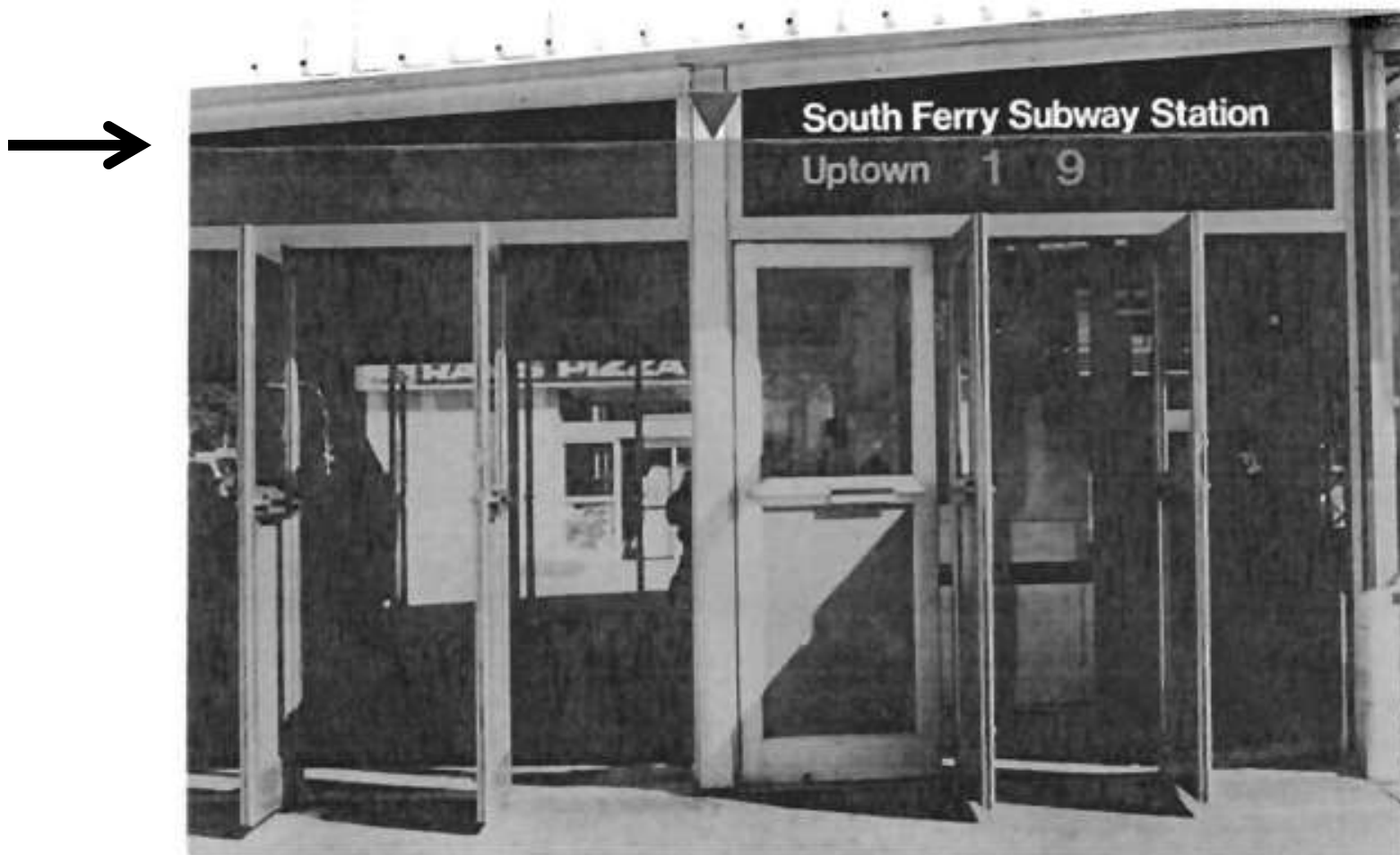
FIGURE 17 - Potential Category 2 hurricane surge at South Ferry (Battery) Subway Station
