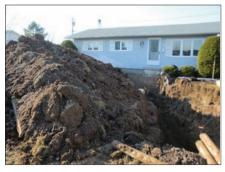
water away from the home quickly; they should never have any standing water. Based on the camera inspection, and before the backwater valves were installed, the laterals had to be torn up and replaced, requiring the excavation of the front yard (See Figure 2).
